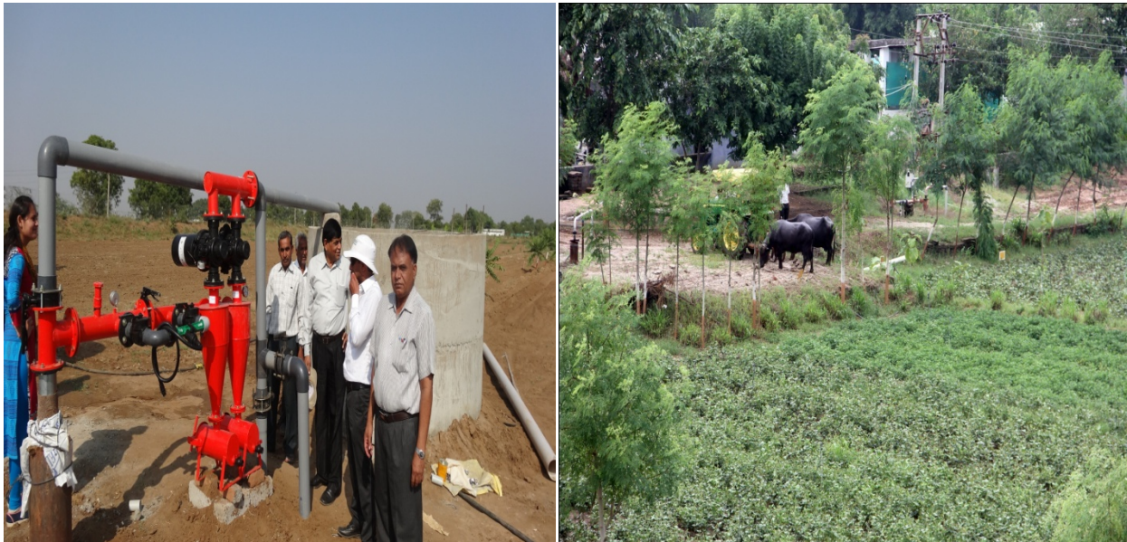
Fig. 4: New borewell dug at IFS farm
